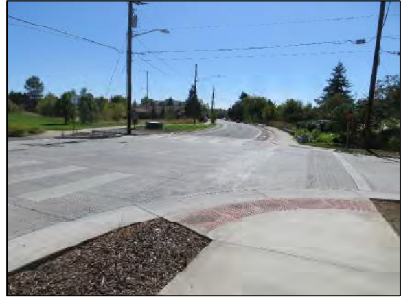
Figure 10: Raised Crosswalk on Oak Street at 14th Avenue in Albany, Oregon
