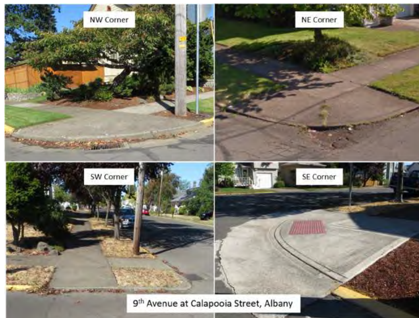
Figure 11: Curb Ramps at the Intersection of 9th Avenue/Calapooia Street in Albany, Oregon
