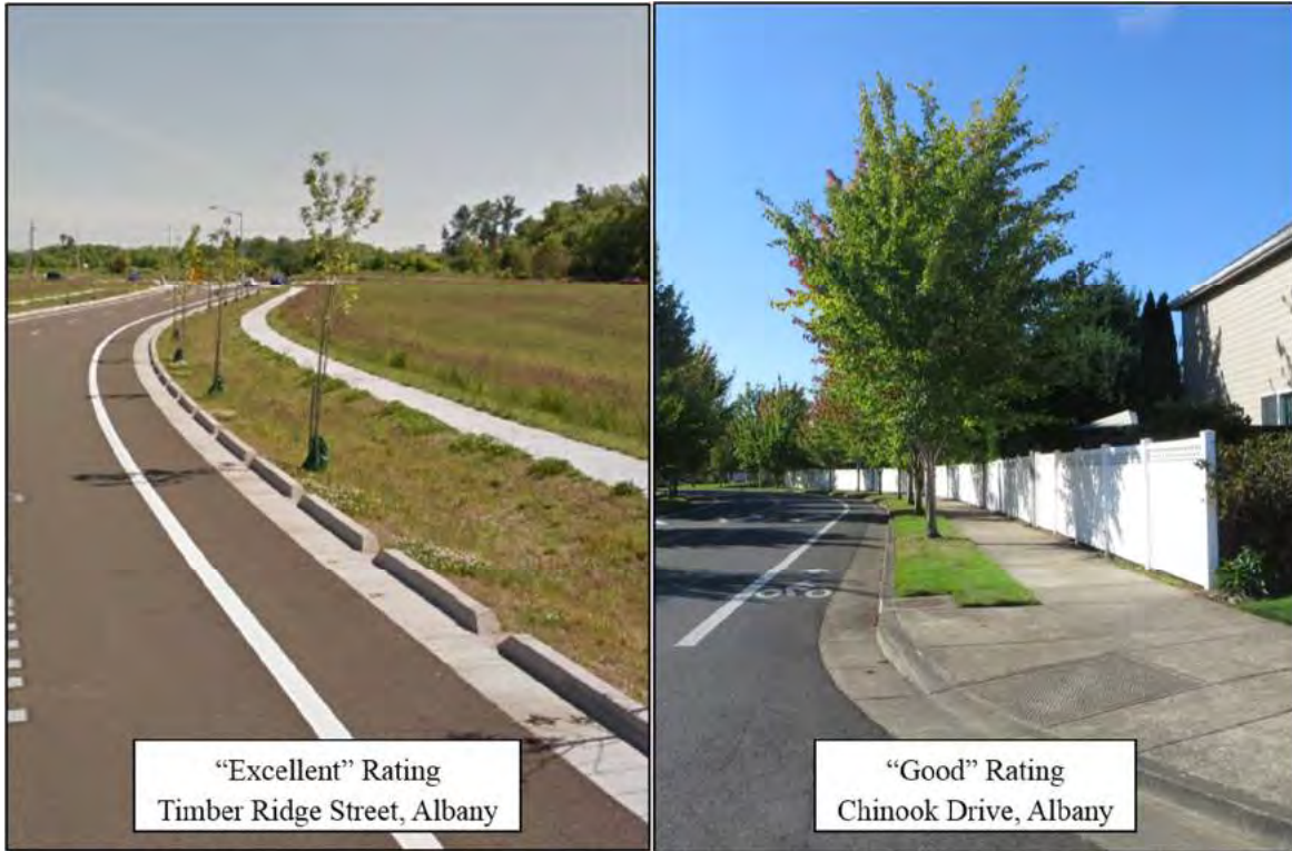
Figure 8: Example of an “Excellent” and “Good” Sidewalk Rating within the AAMPO Area
