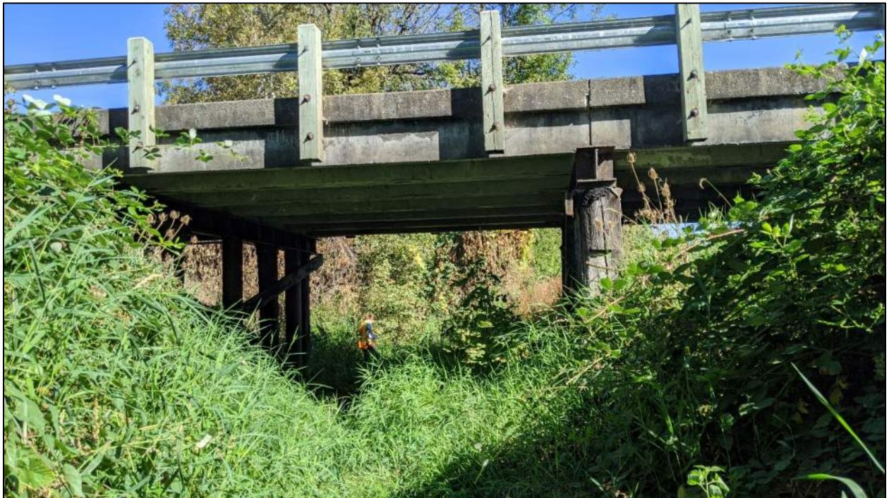
Photo 4. Mill Creek drainage, looking upstream toward the Folsom Road SE bridge.
