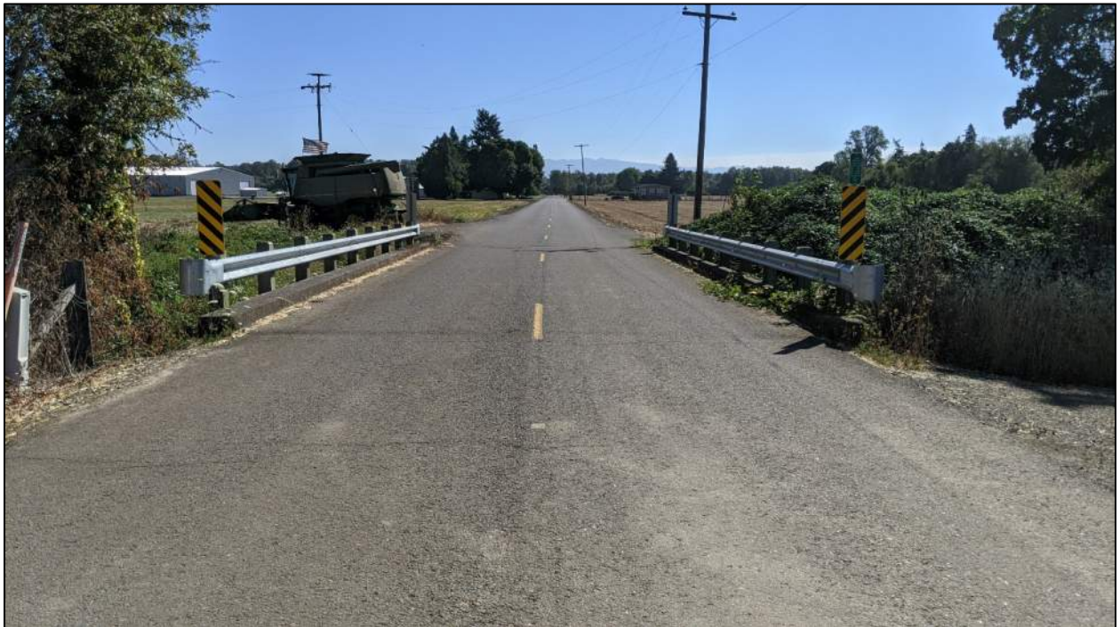
Photo 2. Looking east along Folsom Road SE at the Mill Creek Bridge.
