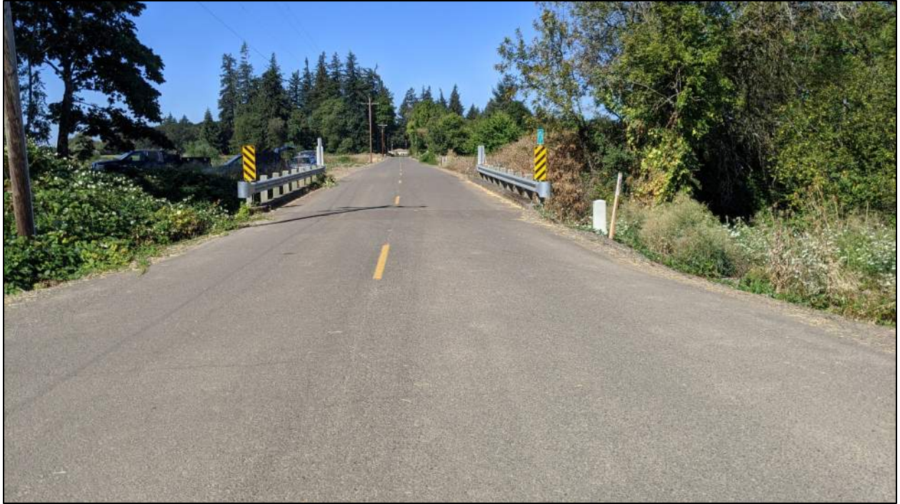
Photo 1. Looking west along Folsom Road SE at the Mill Creek Bridge.
