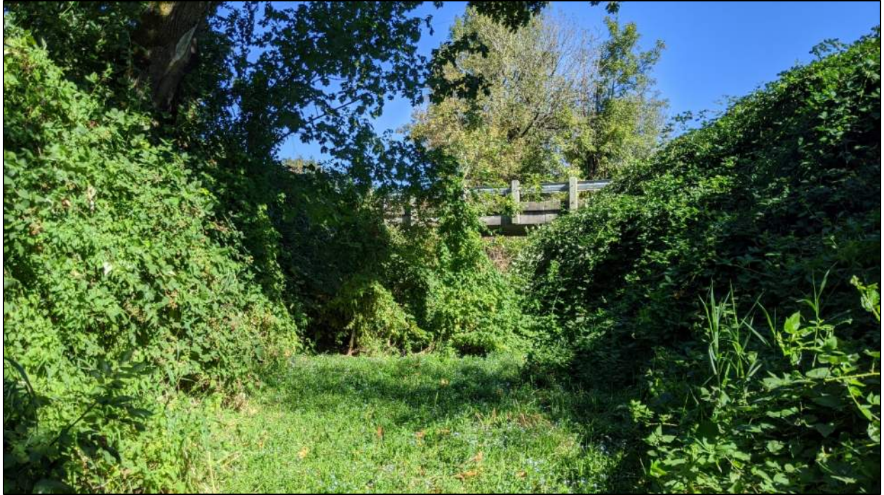
Photo 3. Mill Creek drainage, looking downstream toward the Folsom Road SE bridge.
