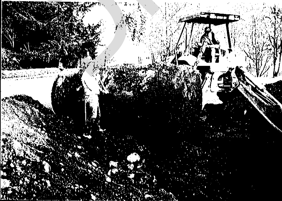
Photo 891208-11 Site Location: North (in front) of service station Direction Faced: Northeast Showing: Tank #2 after removal
