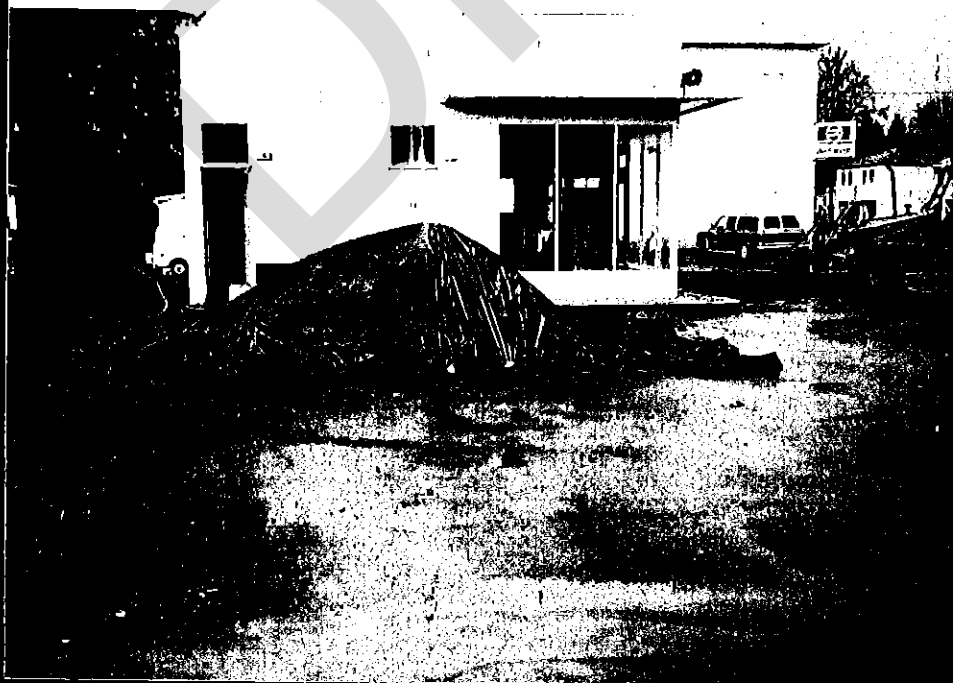
Photo 891209-13A Site Location: East side of site Direction Faced: West Showing: Contaminated soils covered with visqueen
