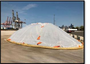
Anchor the plastic using sandbags or other suitable tethered anchoring system spaced on a 10-foot grid spacing.
