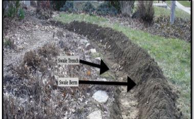
Image 12. Soil Dike with Swale
