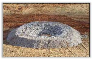
Image 17. Aggregate Inlet Protection
