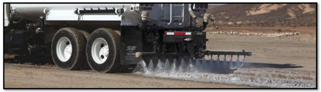
Image 3. Soil Binder Being Hydraulically Applied to Bare Soil
