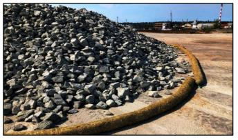
Image 23. Sediment Barrier at Parameter of Stockpile
