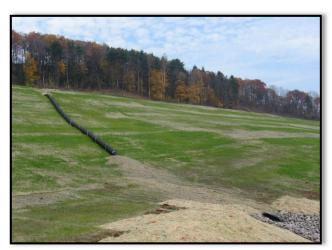
Image 14. Piped Slope Drain with Energy Dissipator
