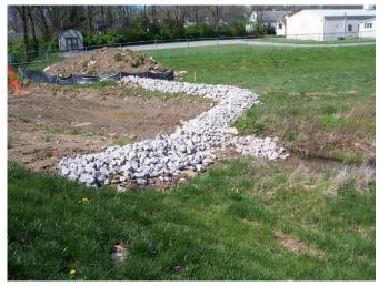
Image 26. Aggregate Filter Berm
