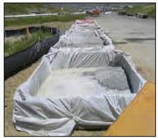
Image 30. Plastic Sheeting Lined Concrete Washout Basin
