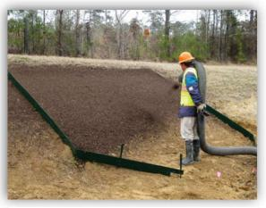
disturbed areas to reduce stormwater runoff and erosion. This material fills in small rills and voids to limit channelized flow, provides a more permeable surface to facilitate stormwater infiltration, and promotes revegetation.
