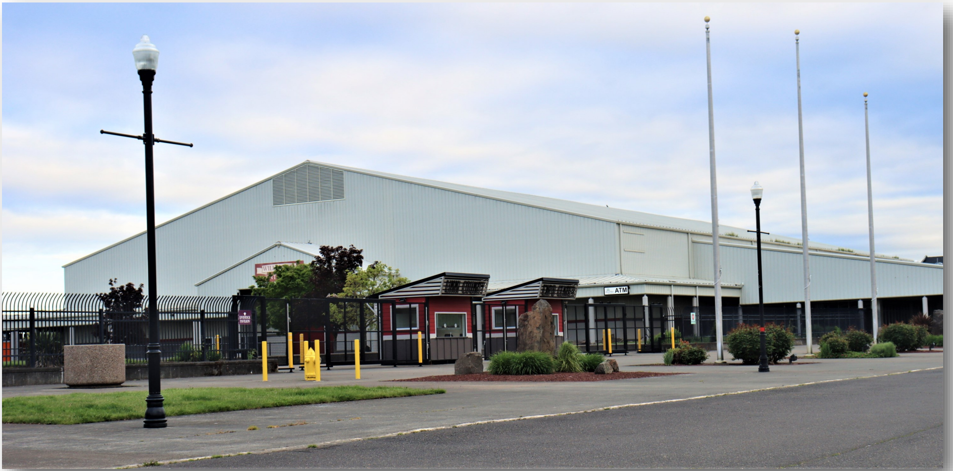
Vendors and others who use the Linn County Fair & Expo Center will see much faster Internet connections due to newly installed fiber optics.
