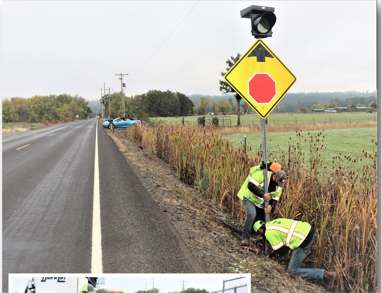
Billy Kelso, Robert Giles and Jarrett Clark of the Oregon Department of Transportation prepare and install a new solar-powered advanced warning flasher on Richardson Gap Road south of the Highway 226 intersection. The driver of the vehicle in the background rolled down her car's window and thanked them for their work.
