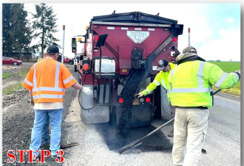
Laying in the 280- to 300-degree asphalt mix.
