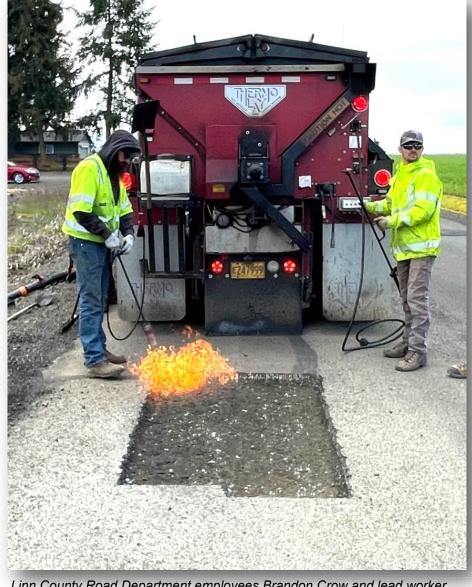
Linn County Road Department employees Brandon Crow and lead worker Mitch Keenon warm up a ground-out pothole in preparation to receive asphalt filling.
