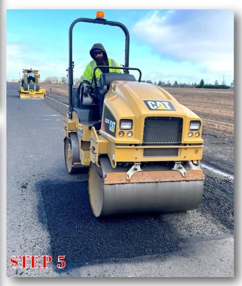
Brandon Crow operates a heavy roller to compact the new asphalt patch.
