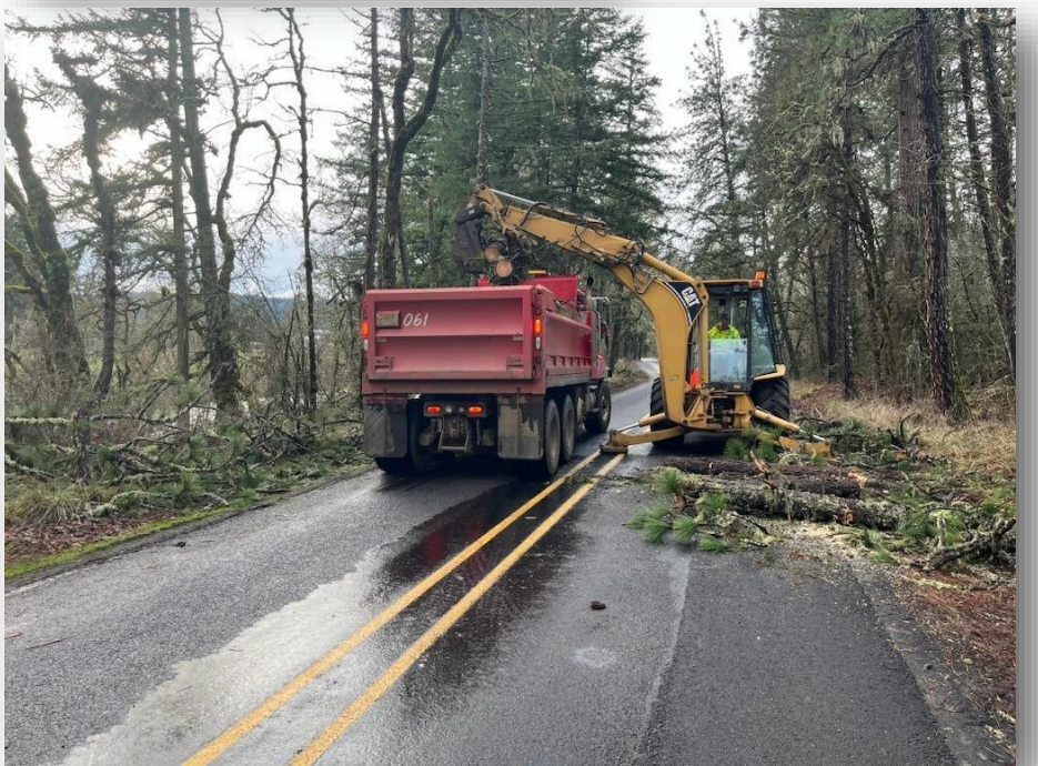
Road Department clearing Crawfordsville Drive.
