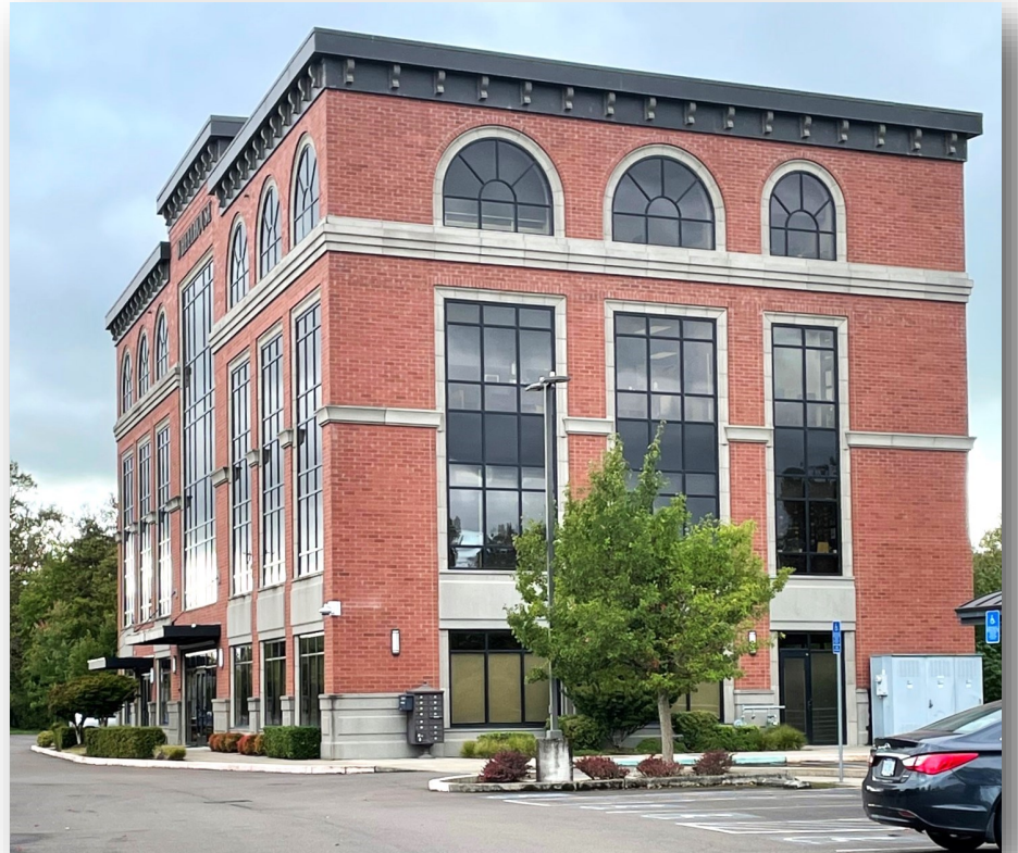
Construction of the Wheelhouse office complex on Water Avenue began in 2008 and the building opened in 2010.
