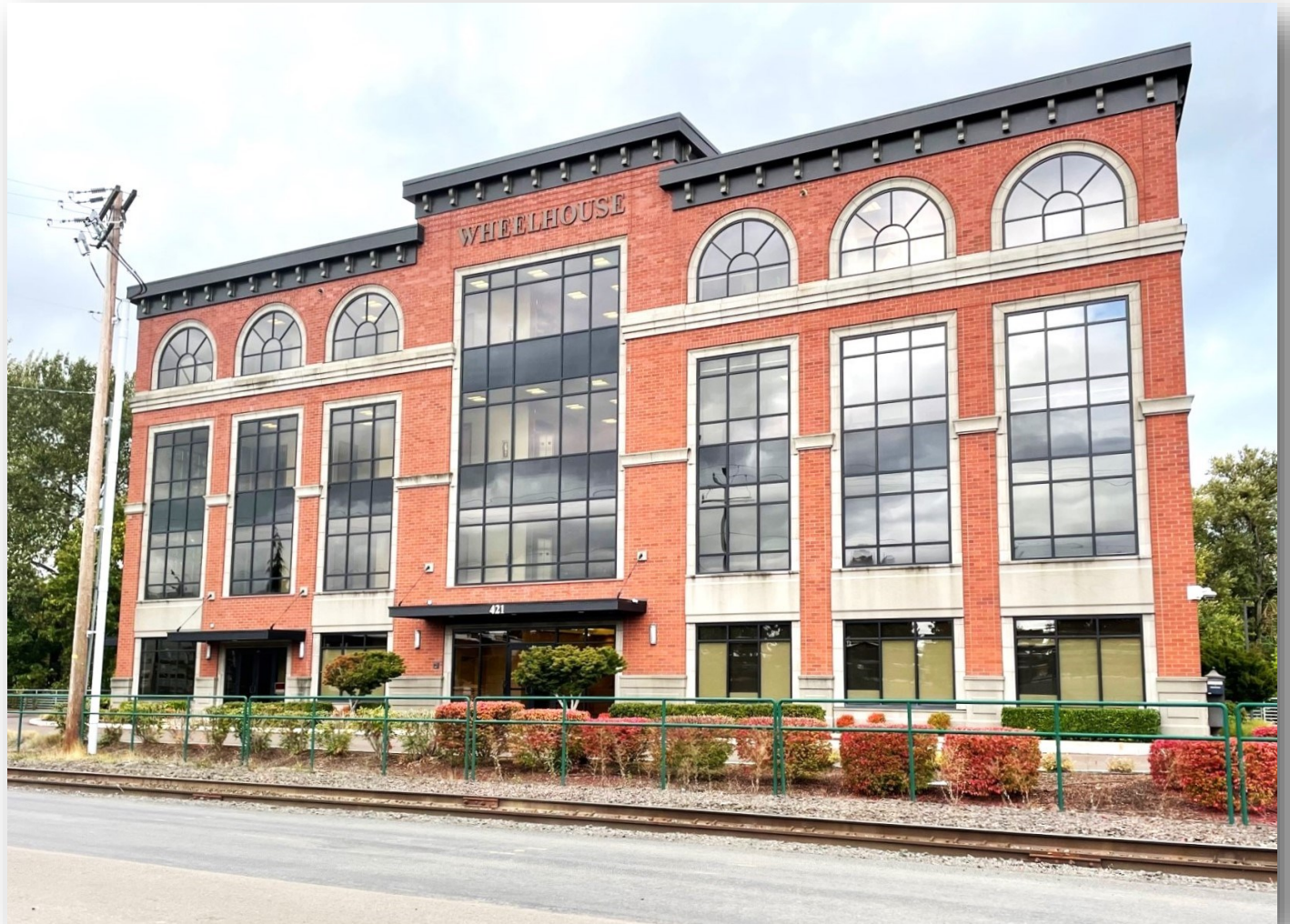
Linn County has begun the due diligence process associated with the purchase of the Wheelhouse office complex at 421 NE Water Ave. in Albany.
